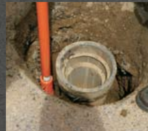
2) Utilize a jack hammer or concrete saw to remove blacktop or concrete around the valve box.
