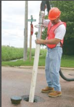
1) Vacuum water and debris from valve box.
