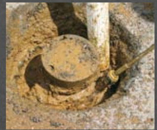
3) The Valve & Vac™ high pressure emulsifying wand sends out a swirling stream of water at 3,000 p.s.i. that easily emulsifies surrounding soil and can be quickly removed with the Valve & Vac's powerful vacuum.
