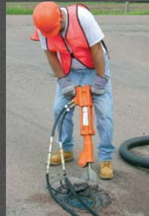
2) Utilize a jack hammer or concrete saw to remove blacktop or concrete around the valve box.
