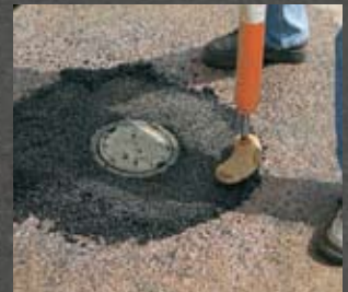
3) The Valve & Vac™ high pressure emulsifying wand sends out a swirling stream of water at 3,000 p.s.i. that easily emulsifies surrounding soil and can be quickly removed with the Valve & Vac's powerful vacuum.
